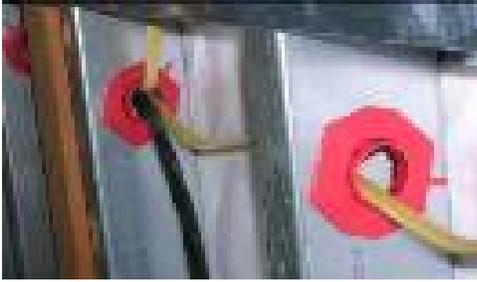
The electrician also noted two products that have improved their efficiency in preventing wires from being damaged as they pull them through steel members. The first one is a plastic grommet that snaps together around the openings in steel studs. These grommets are hard to move and take little time to install. The second product is a
