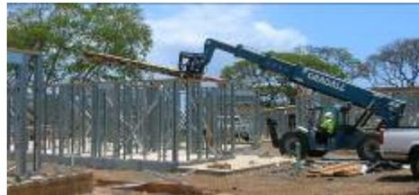
Pictured to the left is a beam with brackets waiting for the forklift to place it on the wall panels and a forklift (above) placing floor joists on wall panels. Notice the placement of the beam on wood blocks to facilitate use of the forklift.
