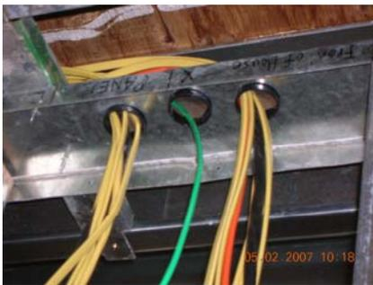
The electrician for the Radford Terrace homes has found working with a hybrid frame that includes steel and wood can require extra effort to run wiring. Although steel wall panels have standardized holes punched in the studs, they do not always end up in a location where the electrician needs to run the wiring. The electrician thus has to cut or drill some studs.
