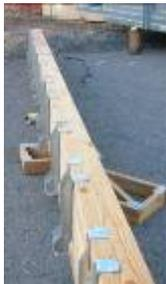
floor wall panels. Beams and joists are set on the wall panels by an all-terrain forklift. During down time the crew preps beams for future installation and helps other crews as needed.
