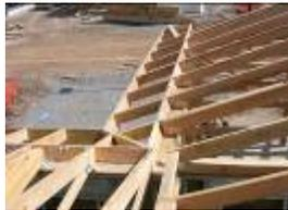
This crew is responsible for attaching the fascia board to the end of trusses. Most of the fascia arrives pre-cut but some modifications are necessary on site. This crew requires tie-off training. Pictured here is the fascia on the truss tails.
