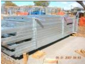
Steel panel wall stacks are stored as close to their desired location as possible when they arrive at the construction site. Wood boxes are used to keep the panels off the ground and enable the forklift to easily get under the panels.
