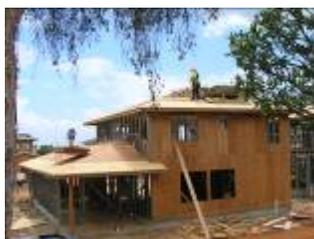
The roofing crew installs the roof sheathing (plywood) after the soffit previously discussed. The crew places a few sheets of plywood that serves as a stand for the rest
