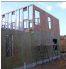
The exterior sheathing installers are responsible for affixing sheathing to the first story exterior walls. The crew also applies brackets to connect first story wall sheathing to second story wall sheathing. Walls that don't require shear resistance are left open. Pictured here is a completed sheathing job.
