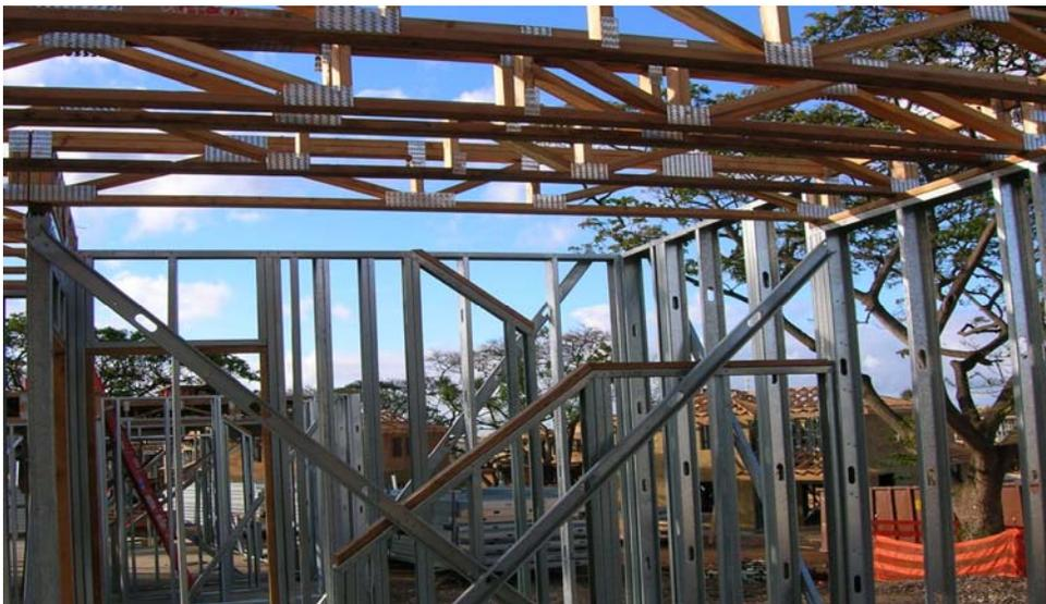
Floor joists supported by steel wall panels. Note that the trusses are each directly located over a stud (inline framing). Further, in order to avoid unusual connection details between the floor trusses and the steel walls, a wood top plate is installed on the panels during fabrication at the panel plant.
