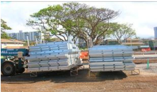
Storage - The necessity for storage makes ample space (land) crucial. Depending on the construction schedule and shipping times, stockpiled panels can take up a vast amount of space. The fabrication plant needs to be ahead of the construction process or else fabrication will slow the construction schedule.
