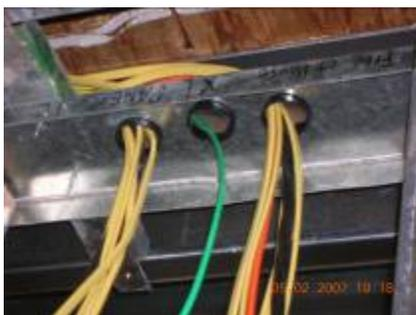
The electrician for the Radford Terrace homes has found working with a hybrid frame that includes steel and wood can require extra effort to run wiring. Although steel wall panels have
