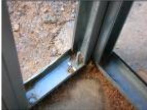
The anchoring task involves installing the permanent foundation tie downs and brackets for high wind resistance and traditional anchor bolts for the first floor wall panels. The crew first attaches brackets to the wall panels. Then they drill holes through the steel panels into the concrete slab. Next air is blown into the holes to remove dust so the epoxy will adhere to the slab and bolt. The bolt and
