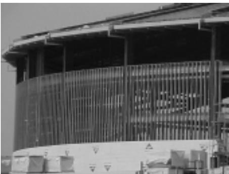
Large curved exterior wall framed with light gauge steel.
