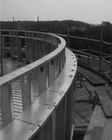
Curved tracks at the parapet tops use both machine-fabricated option on left, and field-fabricated option on right, both approved for their structural capacities.
