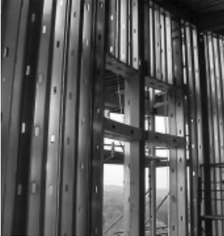
Curved openings using light gauge steel framing, from inside the cupola.
