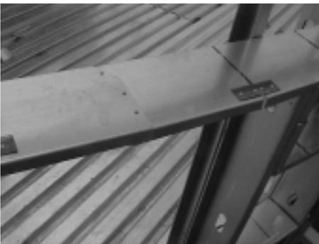
Spliced track at curved parapet.
