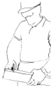
**STEP 3 MARK TRACK:** Lay the top and bottom tracks next to each other in place (on the chalked line) and mark the stud locations.
